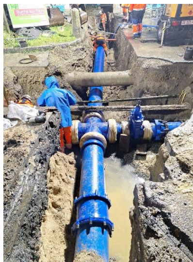
Raccordement surpression Lorette – Rue du Gal Patton
